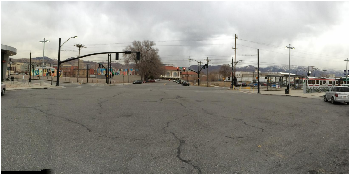
Panoramic view of 300 South from Intermodal Hub (600 West)
