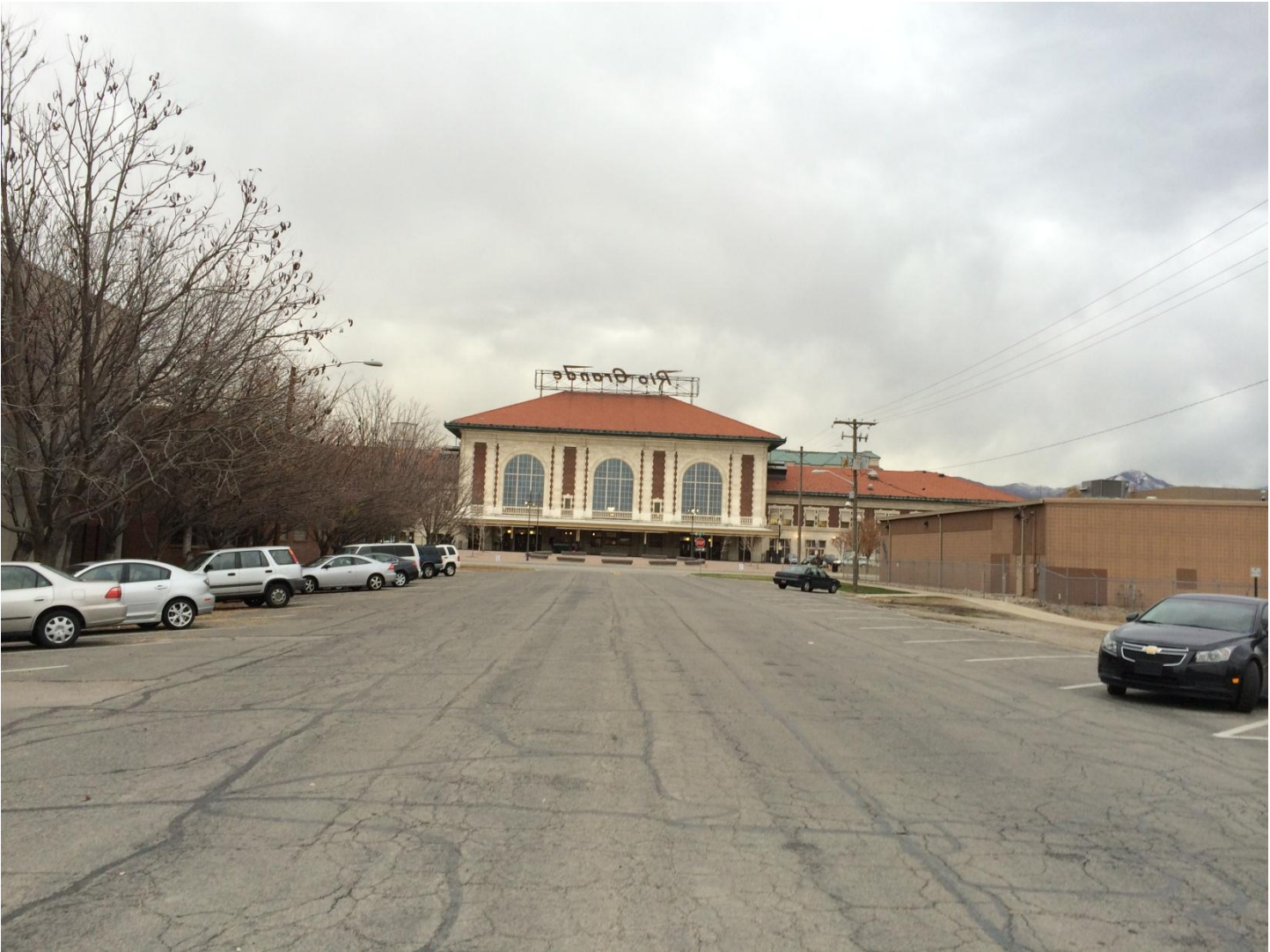
View of Rio Grande Depot from the middle of 300 South
